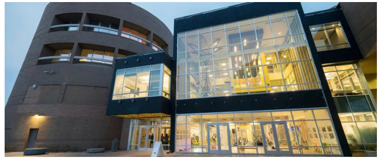
Photo – anchoragelibrary.org – New atrium and entrance of the Z. J. Loussac Library in Anchorage.
