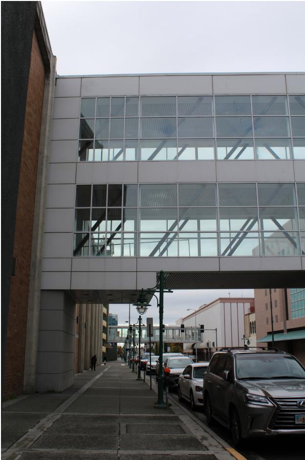
Photo – Planning Department 2020 – 5th Avenue at C Street.
